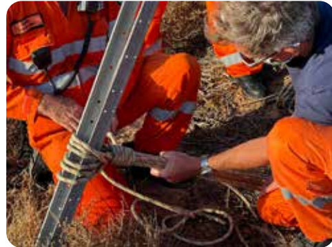
Photo left: Close up of Anchor point. A two person job to secure the ropes tightly.
