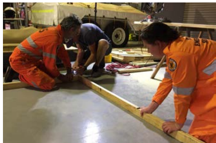
Measuring.... Cutting... Fixing...
